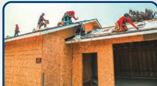
Safecover Roofing ROOFING
